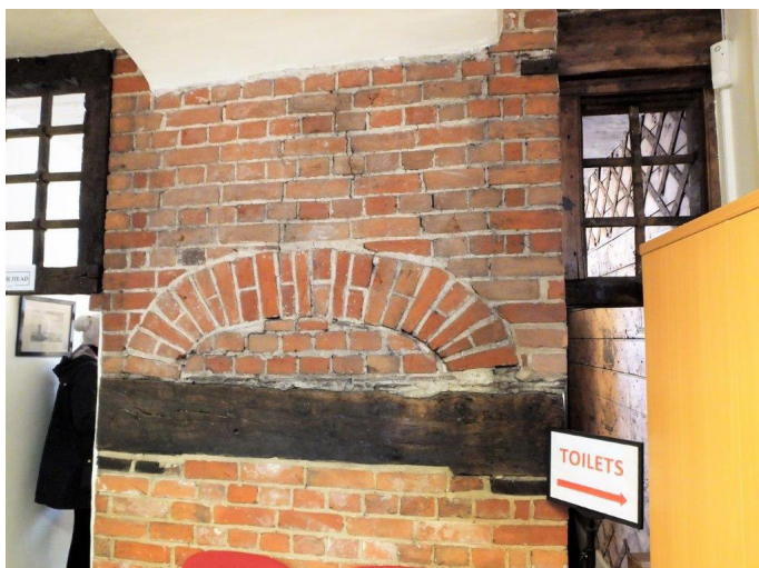
Pine frame visible in entrance hall. Wall is division between cross wing frame and hall
