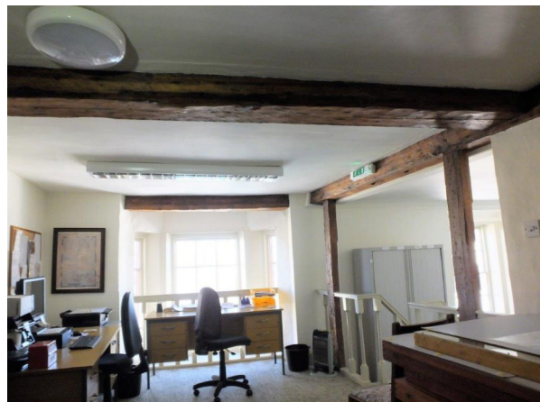
Pine frame visible in entrance hall. Wall is division between cross wing frame and hall
