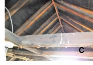
bridled scarf joint in wall plate. C – View to upper roof showing softwood rafters and ridge board. D – Typical side view of roof with added timbers to support plaster.
