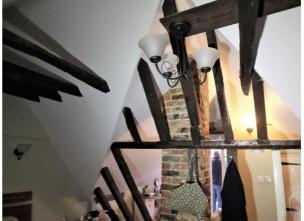
The original form of the pine roof has been altered to allow access to a later rear extension. This has left exposed the empty square mortises in the top of the rear wall plate where the common rafters would have been set. Diamond set ridge with collared rafters to house the purlins.
