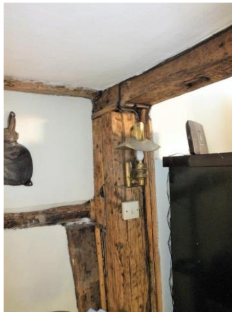
Timbers inserted for the roof raise
