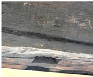
Window mortises at front and axial beam with crenellations
