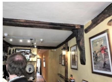
Window mortises at front and axial beam with crenellations
