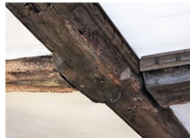
Window mortises at front and axial beam with crenellations
