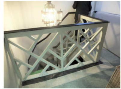
Simpler form of balustrade when modified to gain access to the rear extension.
