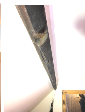
quarter mast section as purlin. Original cut out for collar before ceiling raise
