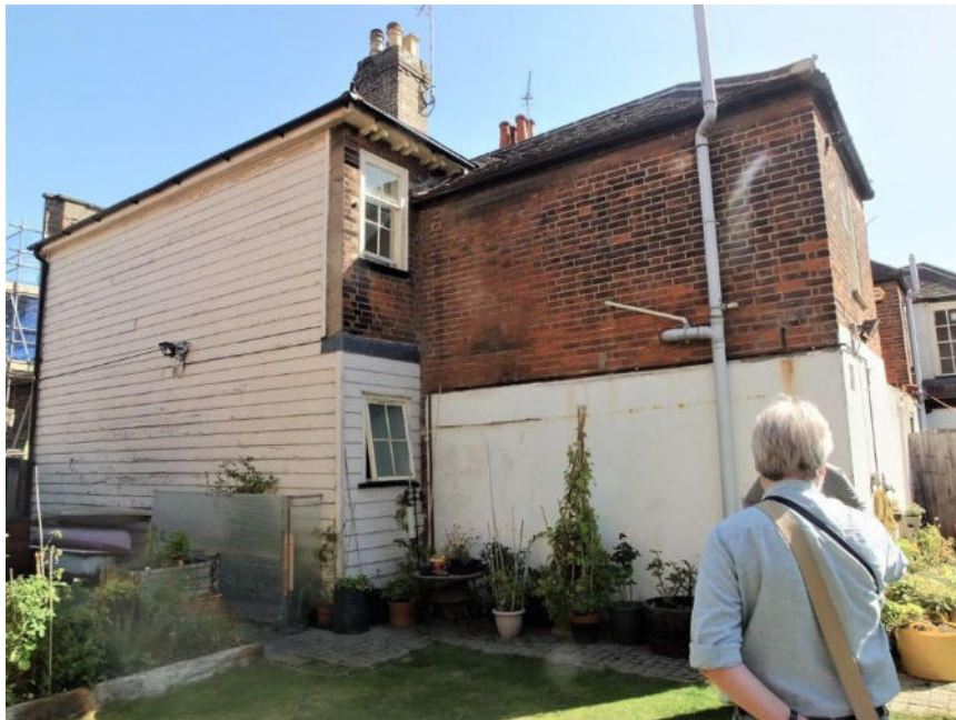
Rear of No.39 showing timber wall and changed roofing detail following removal of chandlery
