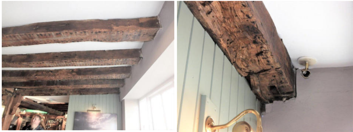
Floor joists of cross wing to street. Jetty plate would have been above the light. Second picture shows remains of mortise for a jetty bracket and mainly destroyed dovetail housing for the jetty plate.
