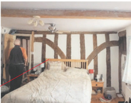
Example of the unusual form of the wall bracing found in the rear range
