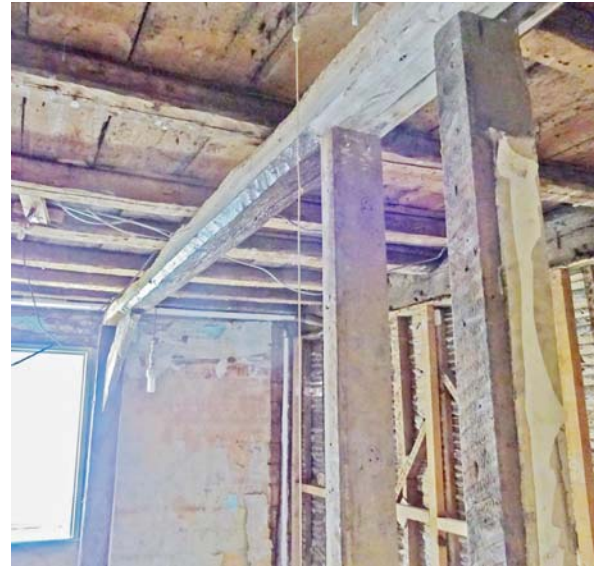
Plate 20 Refixed headbraced crownpost (against far wall) and associated collar-purlin
