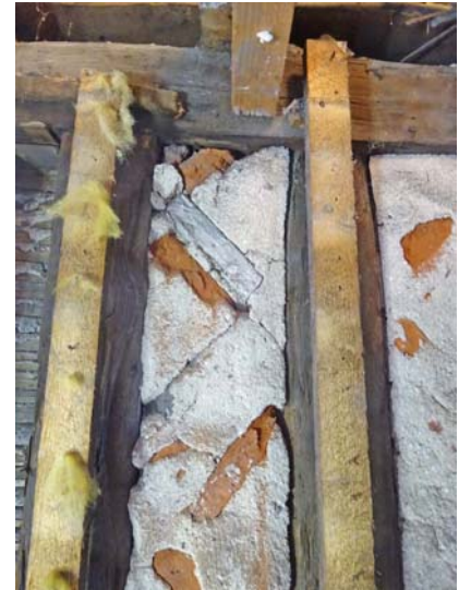
Plate 10 Brick infill to front wall, first-floor level
