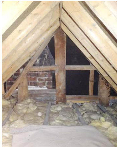
Plate 5 Fragment of rear (east) roof gable of north crosswing visible in gable of modern roof
