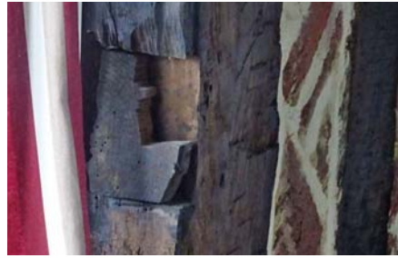
Plate 25 Joint for cill of oriel window, front wall of bay J-K
