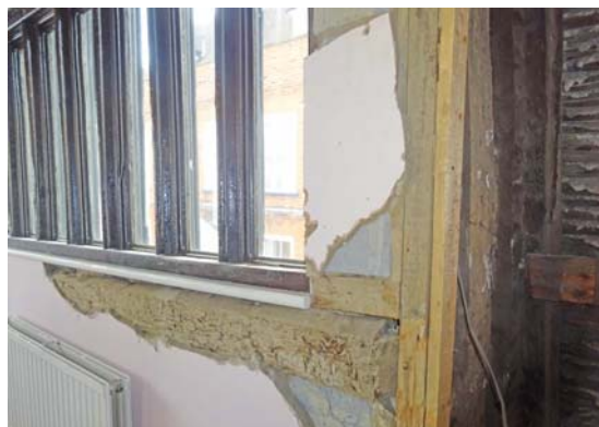
Plate 36 Northern end of west wall showing cill halved and nailed to side of stud in south wall of south crosswing
