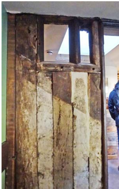
Plate 24 Surviving section of clerestory window, close studding and plastered brick nogging in rear wall of bay J-K
