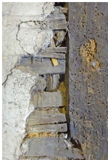
Plate 11 Daub infill on ground floor of north wall, viewed internally
