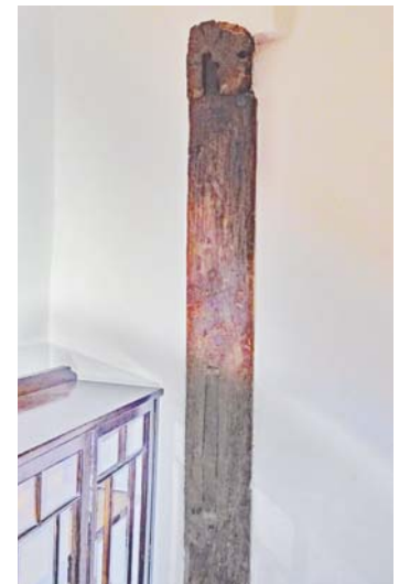
Plate 3 Principal post C in north wall showing cut-off tiebeam and mortice for former arch brace
