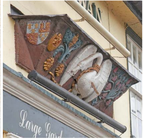
Plate 15 Cill of an oriel in Clare, Suffolk, similar to that which formerly existed in the front wall of the crosswing
