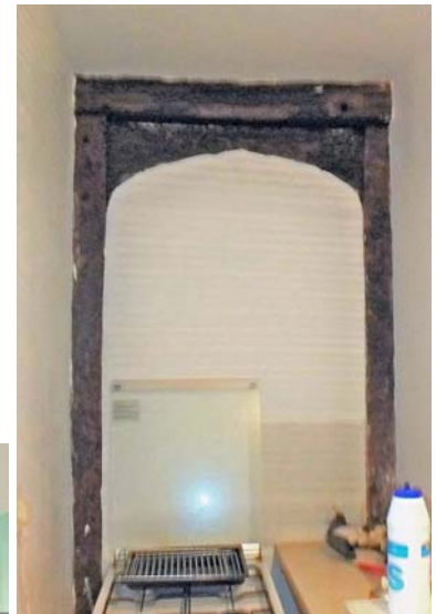
Plate 27 Western end of south wall, north crosswing: inserted period-D1 doorway with arched head replacing plain square-headed doorway of period-B date on same site
