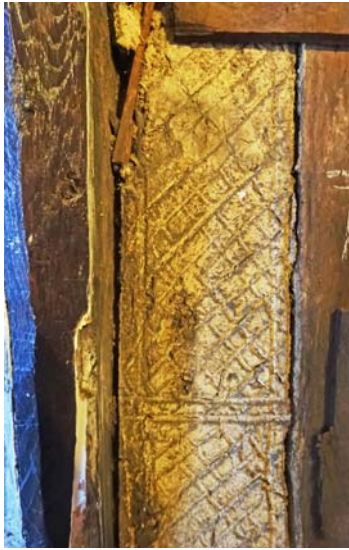
Plate 13 Incised pattern on face of first-floor panel, north wall viewed internally
