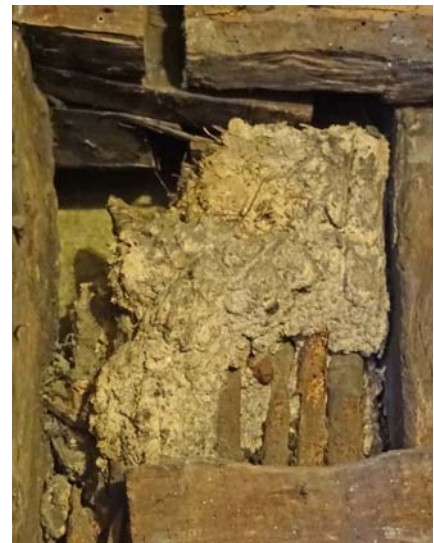
Plate 12 Daub infill on first floor of north wall, viewed internally
