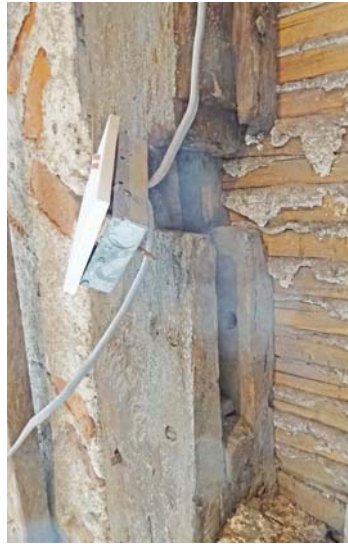
Plate 14 Mortices for cill of former first-floor oriel in front wall of crosswing
