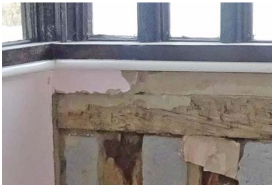
Plate 35 South-east corner on first floor showing chamfered top to window cill with the sawn-off corner post at the extreme left-hand end of the wall
