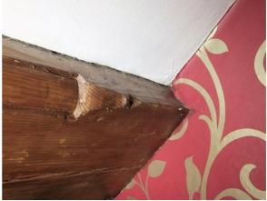
typical 17<sup>th</sup> century end notch. Common joists, also in softwood are of square section and housed with soffit tenons. Many appear to be reused and not matching pre-cut tenons in main beams.
