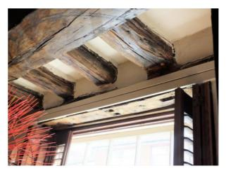
The first floor contained a single chamber with heavy braces from unjowled storey posts of the central truss. Traces of green paint were detected in the front bay. The roof structure has been completely rebuilt to accommodate an attic.
