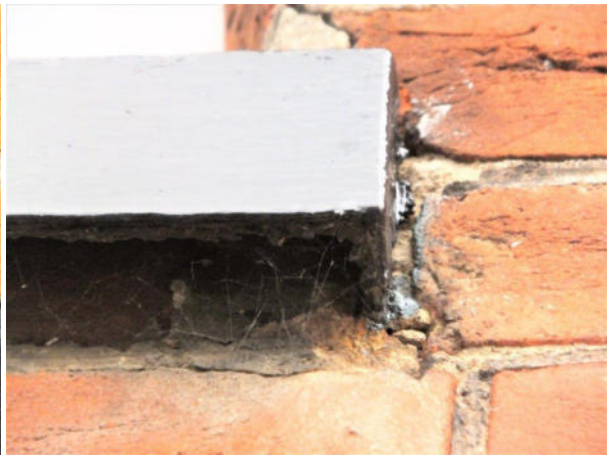
View up under sill to show hollow casting.
