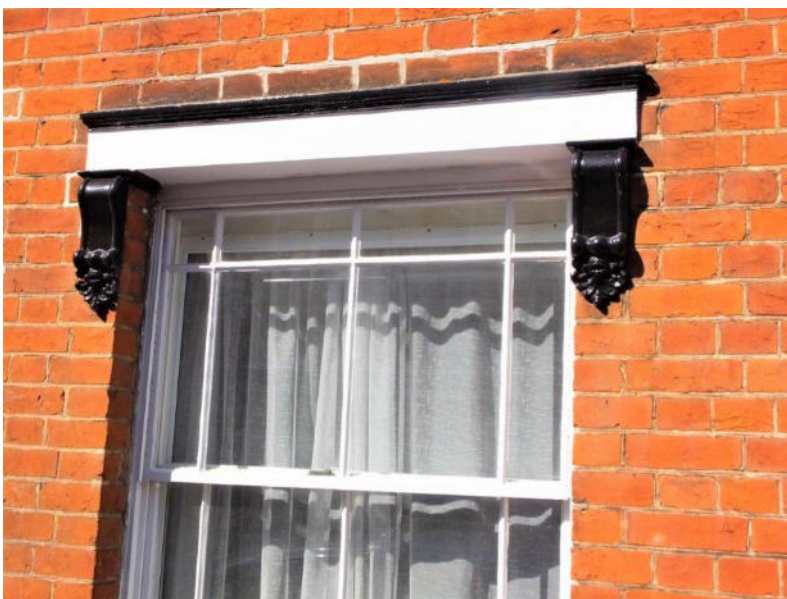
Console bracket in cast iron supporting a cast iron head to the window plate.
