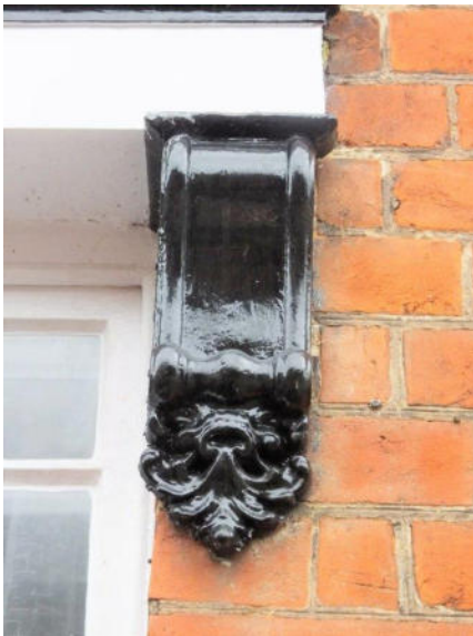
Console bracket in cast iron supporting a cast iron head to the window plate.
